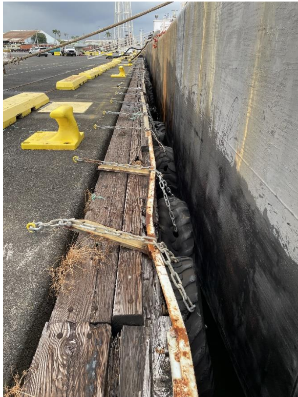
Photo 6: Existing Pier 3 to be repaired. View looking southeast.
