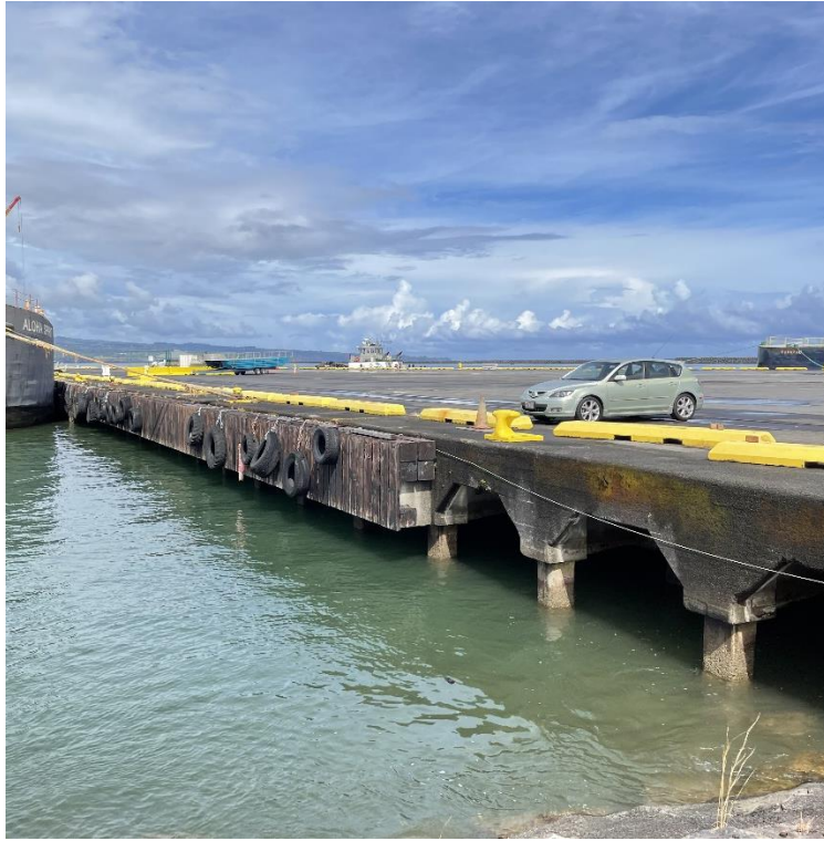
Photo 1: Existing Pier 3 to be repaired. View looking north.
