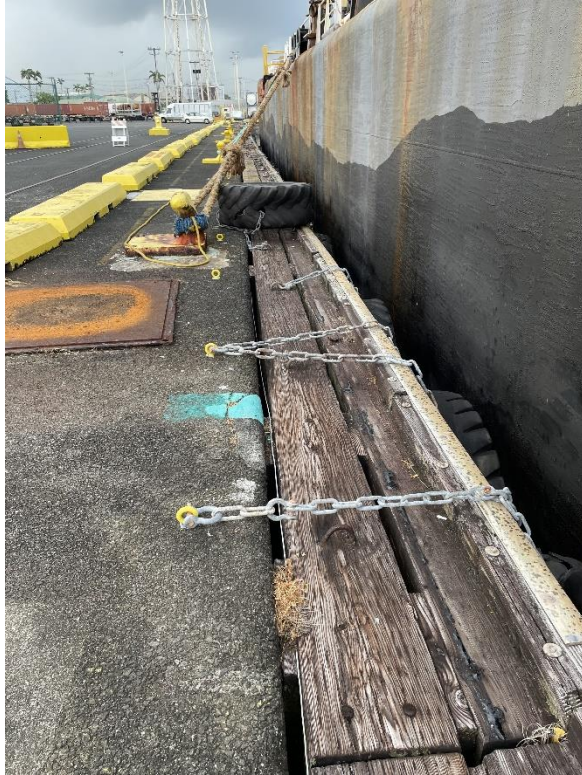
Photo 5: Existing Pier 3 to be repaired. View looking southeast.
